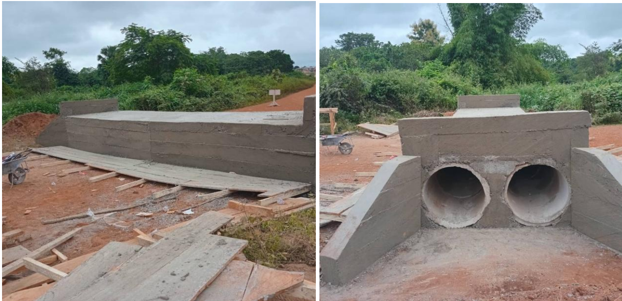
CULVERT AT KOKOSUA
