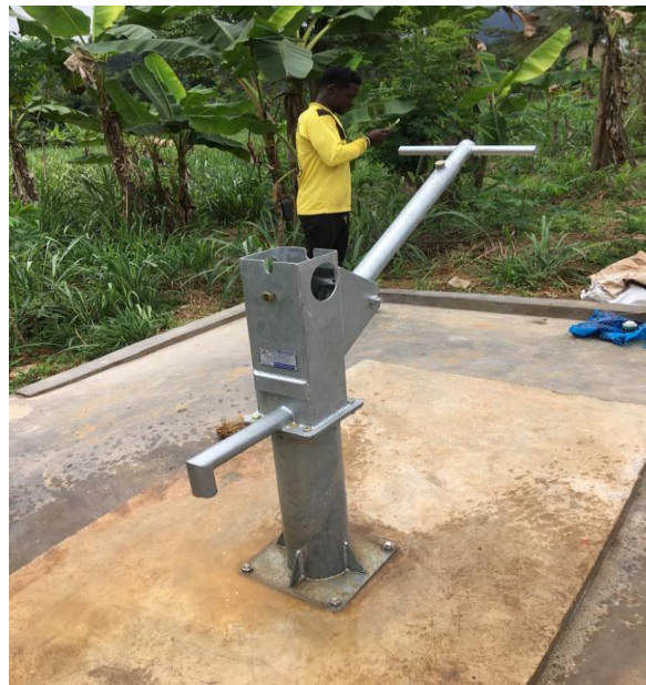
Borehole with hand pump at Suma-Ahenkro-(DACF-RFG)
