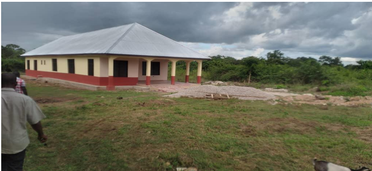
Constructed a maternity block at Goka (DACF)
