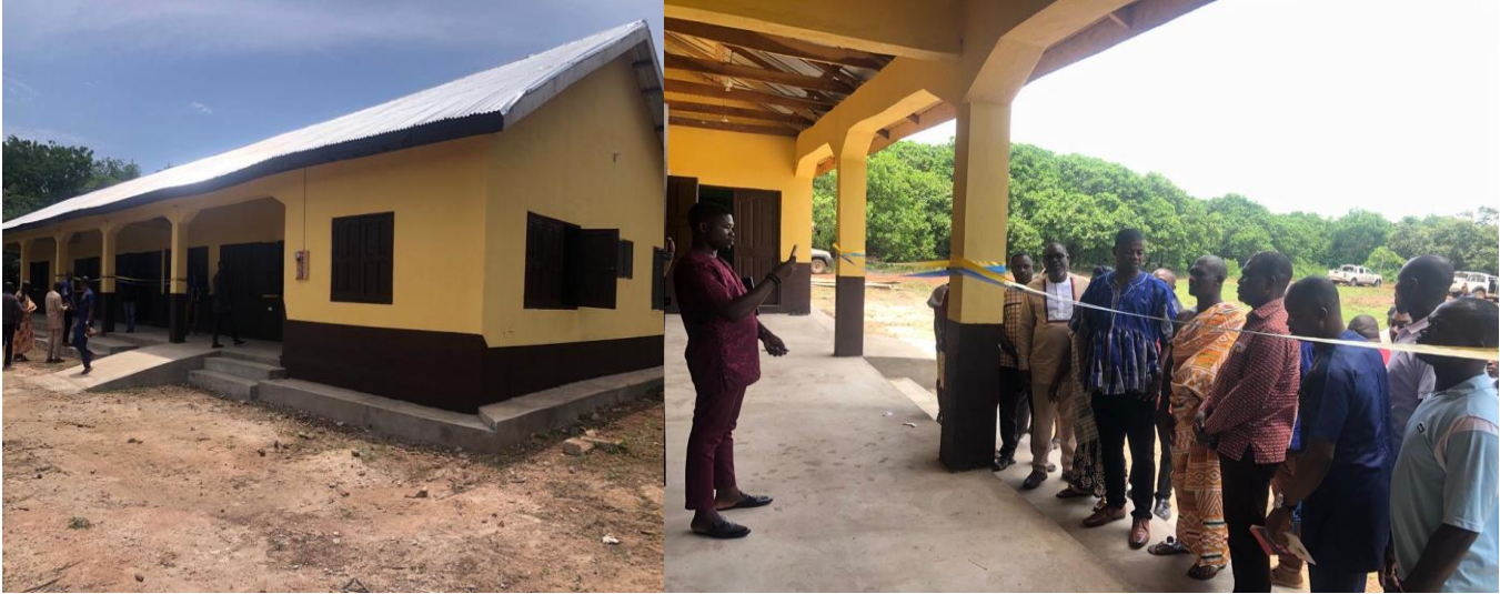
Constructed 3 Unit Classroom Block at Adinkrakrom (DAFC)
