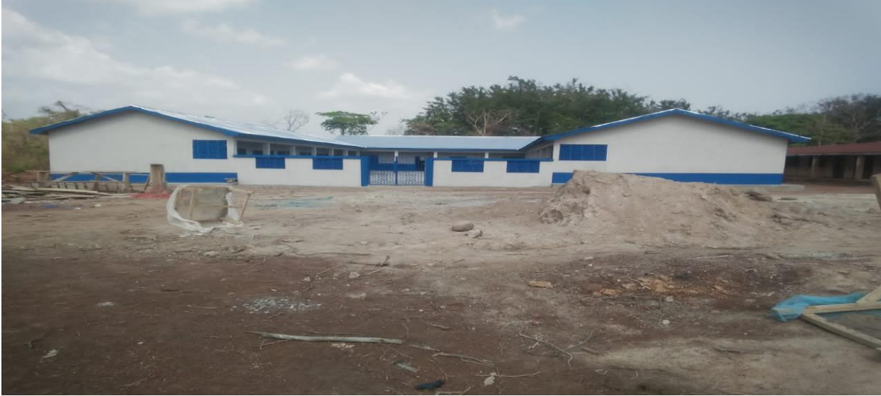
Constructed a 6 unit classroom block and staff common room at Jankufa Presby school (DACF-RFG)
