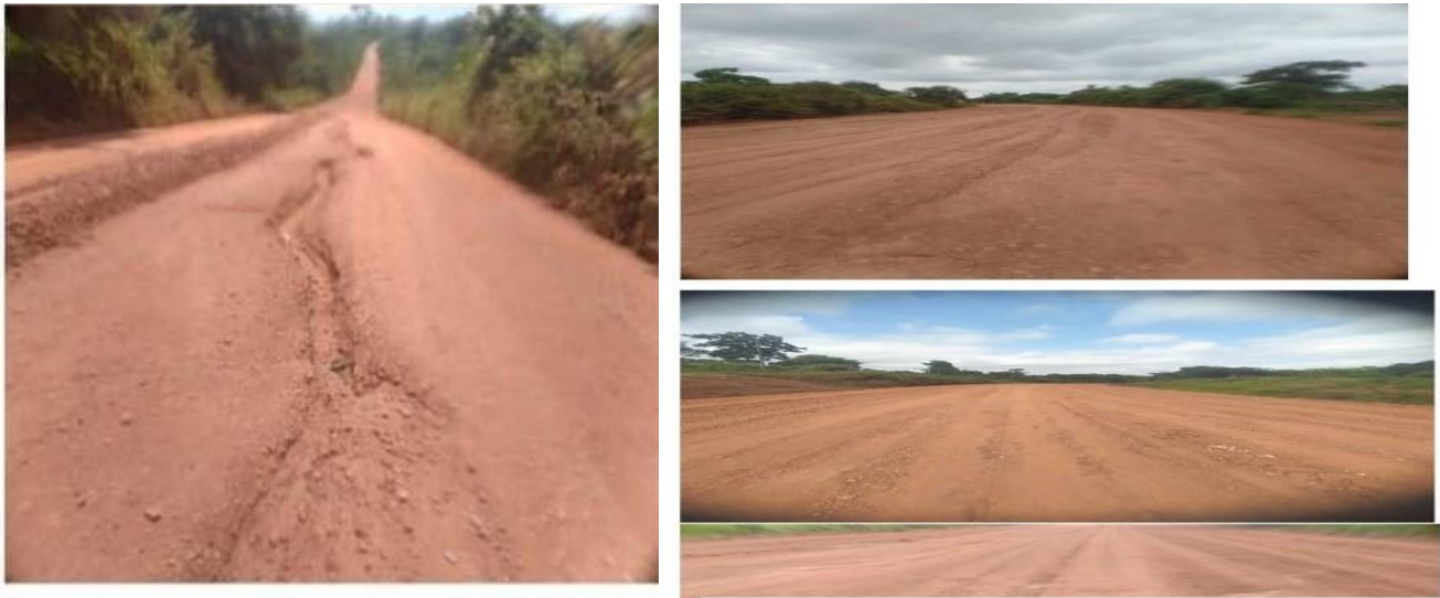
Scarified and compacted Ponkor Junction to Sampa Road (IGF)
